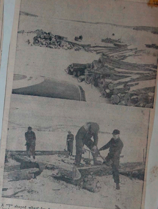
That's a wind sock for aircraft in the distance. BOTTOM PHOTO, foreman Gordon Samuels, North Bay, holds a log steadily while it is drilled by Harold Smith, North Bay. The wharf will be 130 feet out from the shore, have a "T" bar measuring 68 feet from end to end. Width of the wharf will be 15 feet. Most of the cribbing will be completed by the break-up time.
