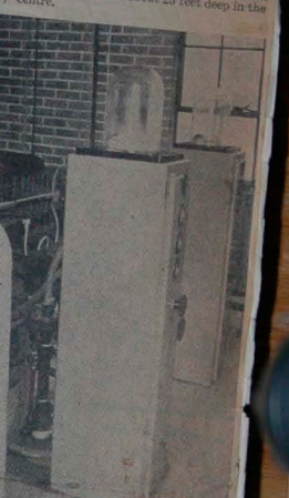
Twin chlorinators inject bacteria-killing chlorine into water entering the pumping station at a constant rate.
