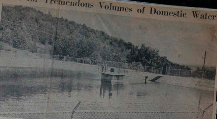
With a capacity of more than 4,000,000 gallons, this high level storage basin atop Reservoir Hill overlooking Trout Lake can be called upon to supply additional sources of water during peak consumption periods.
