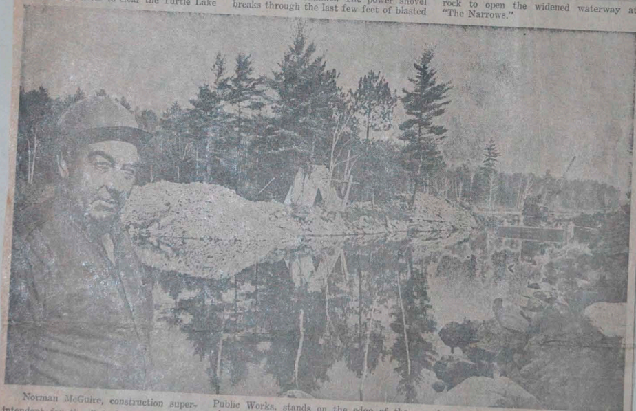
Workmen prepare to drill the last set of dynamite holes to clear the last section of the channel. The power shovel breaks through the last few feet of blasted rock to open the widened waterway at "The Narrows."
