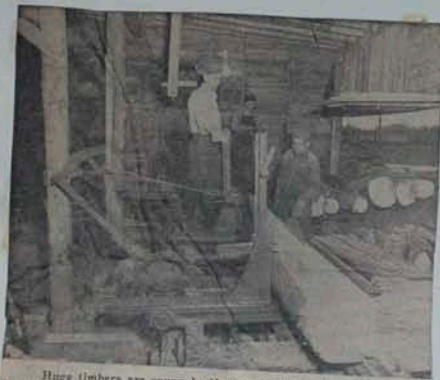
Huge timbers are squared off and cut into lumber. The sawmill is all electric and has a capacity of 10,000 board feet per day. Employees are all skilled and reside in North Bay and district.
